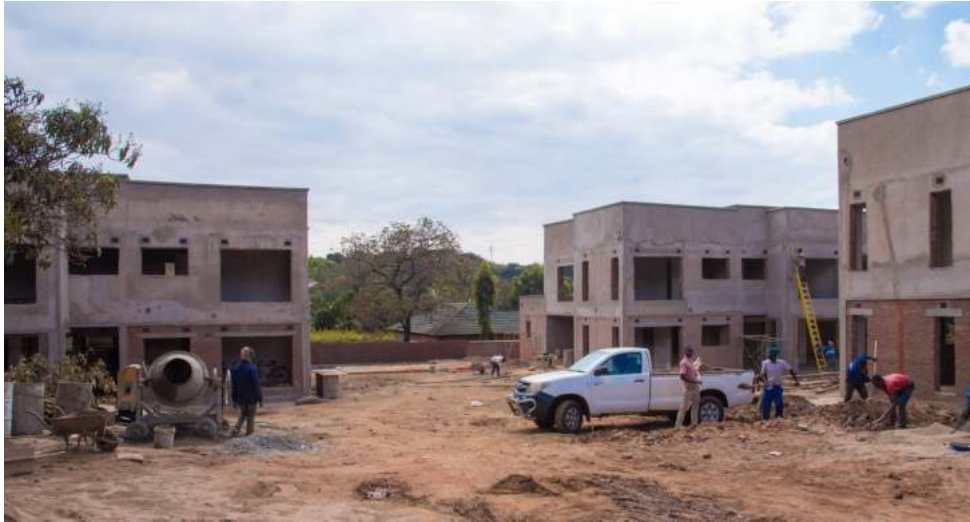
Apartments in Lilongwe City under construction by Mdoko.
