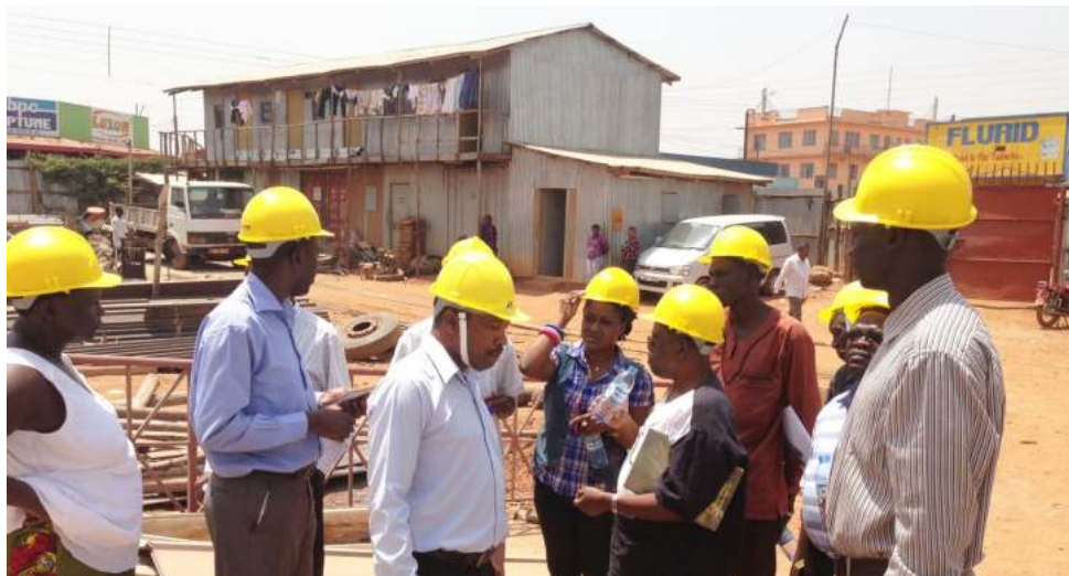
Nnaggenda-Musana checks works on site.
