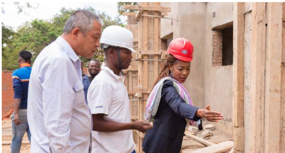
Mdoko supervising construction works.
