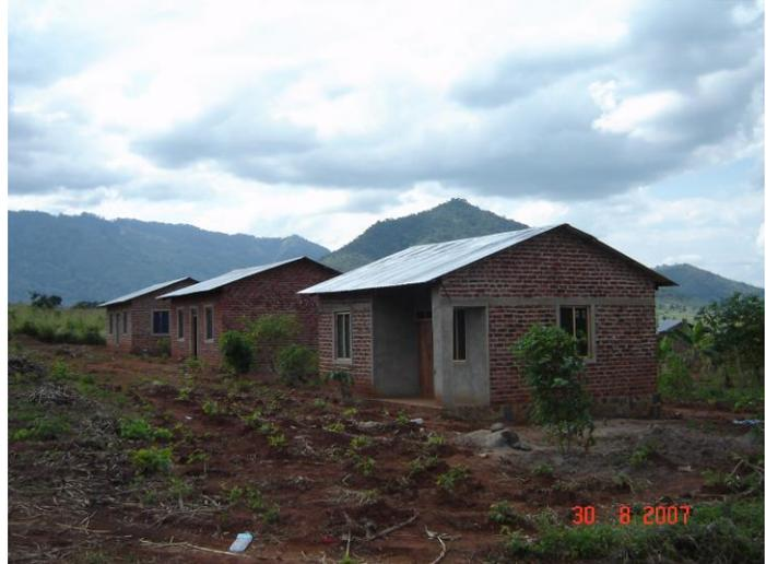
The work was demanding. Completing three houses in two weeks is a challenge. The three house owners got the project started on the right foot by having the foundations laid before we arrived. The families dug the foundation trench and filled it with stones, which are readily available in the area. This left our volunteer team to begin our work building walls using burnt bricks and sand cement mortar. After
